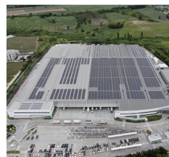
Ricoh Manufacturing (Thailand) Ltd.の社屋屋上
