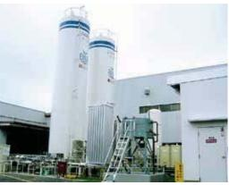
Exterior of the cogeneration system: Liquefied natural gas tank (left) and gas engine power generator building (right)
