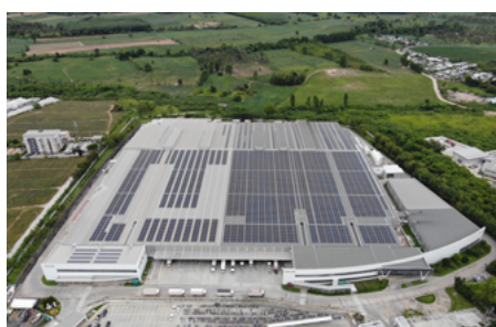
Ricoh Manufacturing (Thailand) Ltd の社屋屋上
